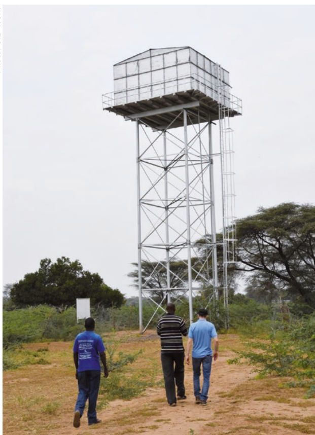
Storage tanks – as funded by WSTF – help to avoid rationing of water supply to low-income areas.
